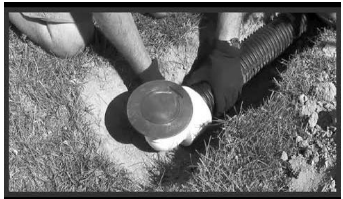
Pop-Up Drain Valve Termination
