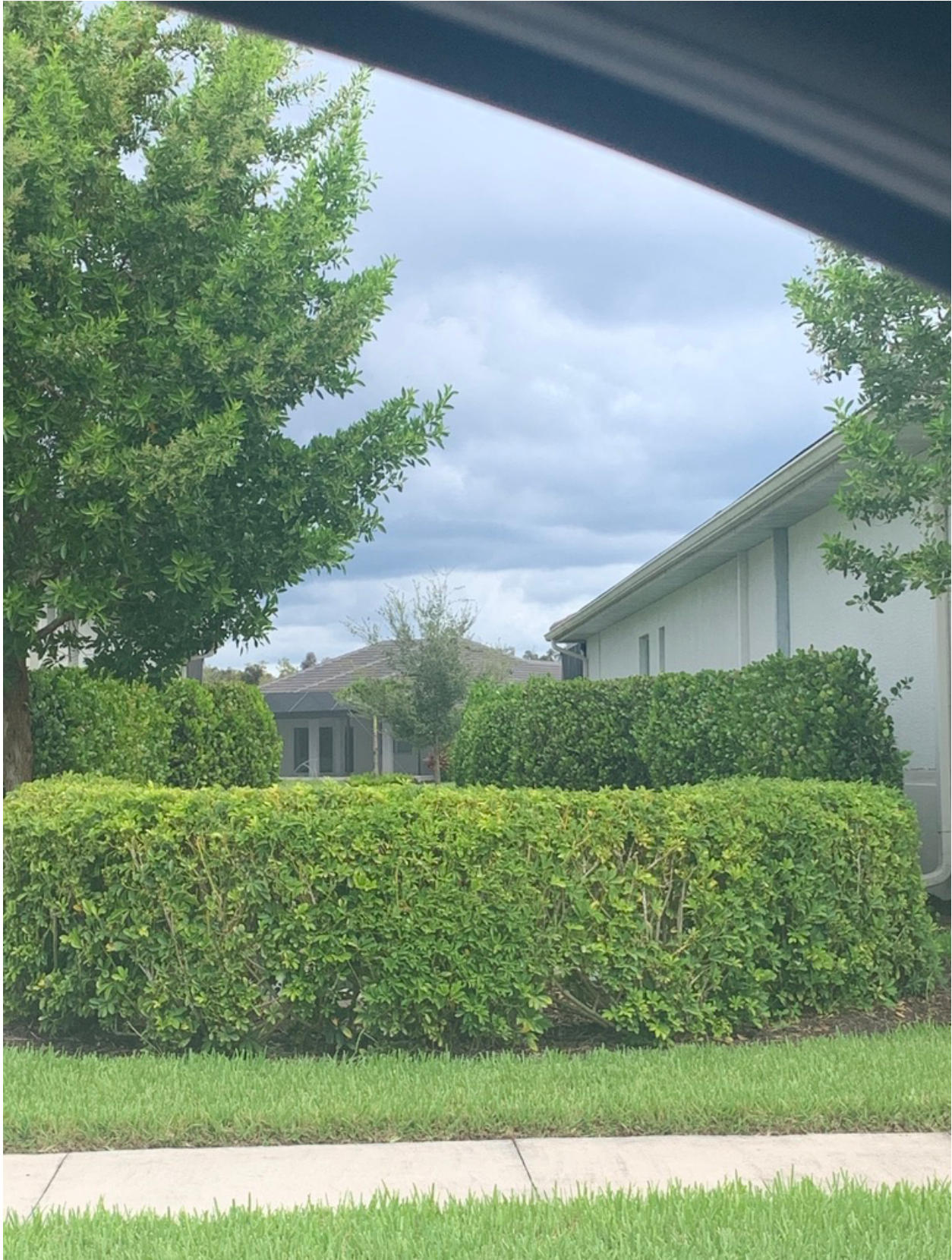
Fig. 13: Between 14311 & 14307 Neptune Ave (Transformer)
